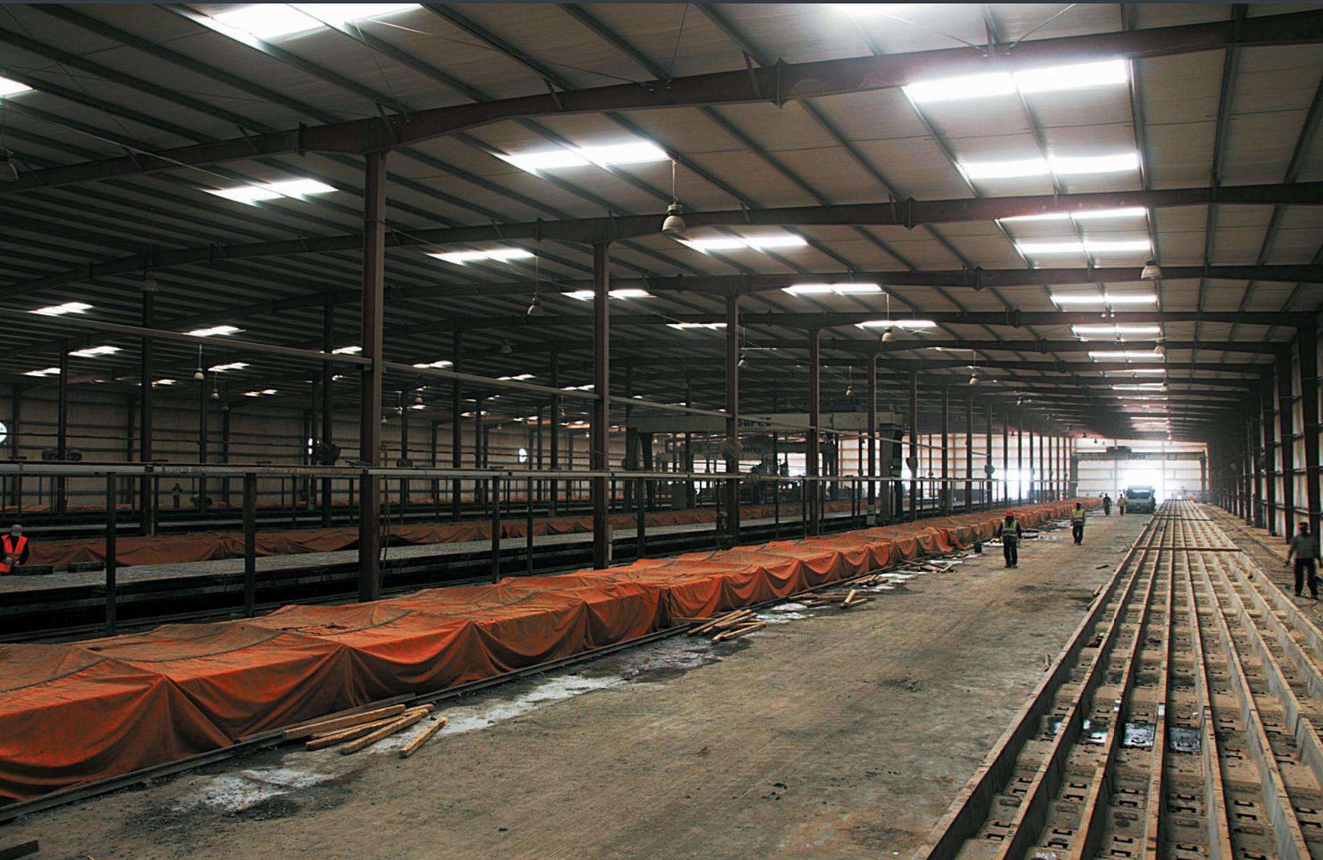
Inside view of factory shed
