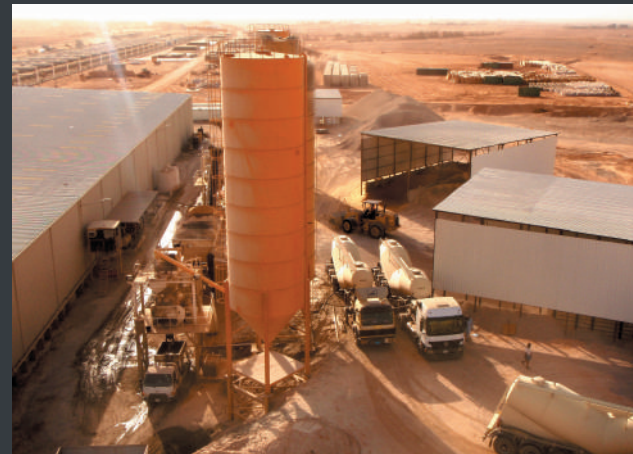
Concrete batching plant
