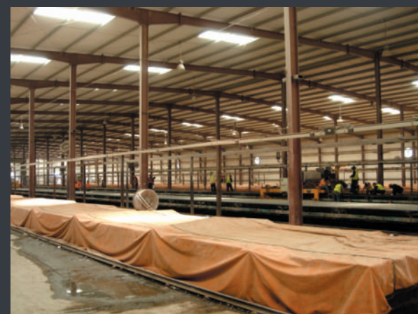
Steam curing of the Sleepers
