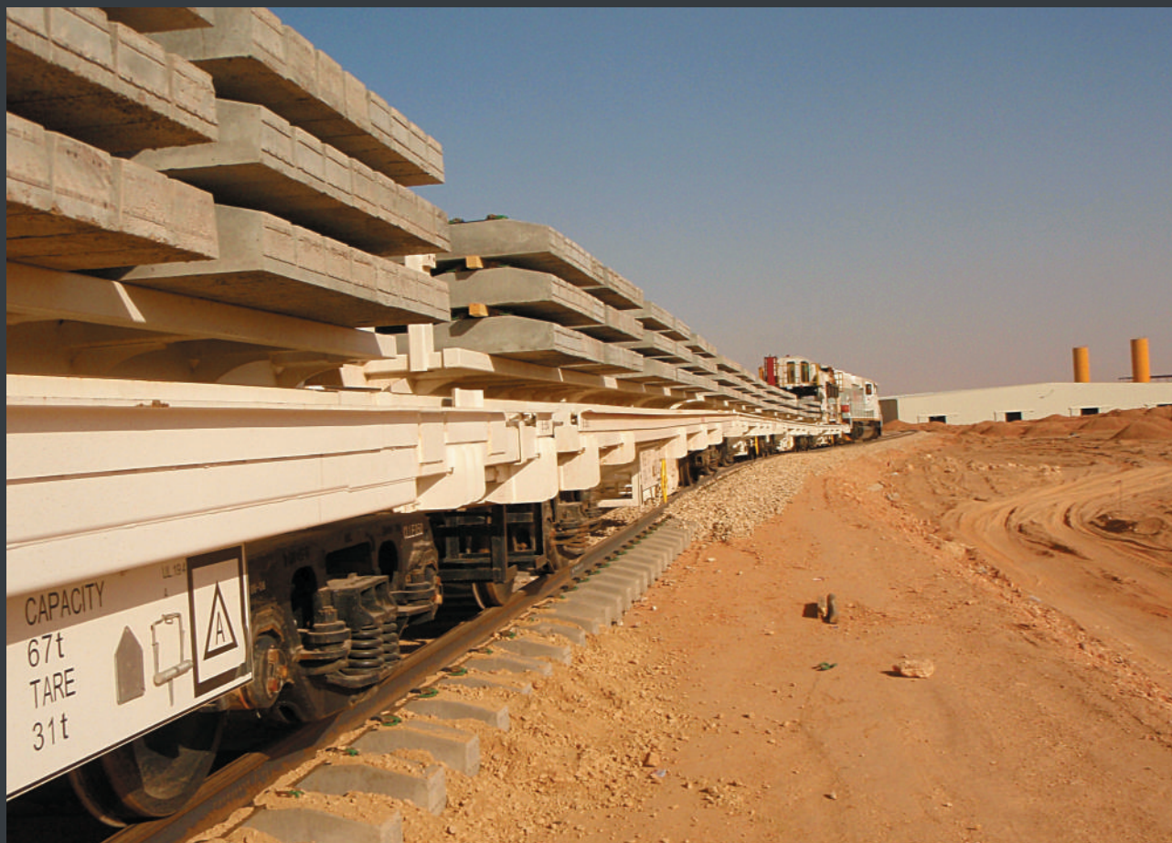
Sleepers dispatch for laying
