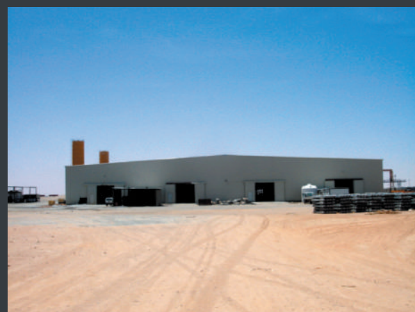
Overview of factory shed
