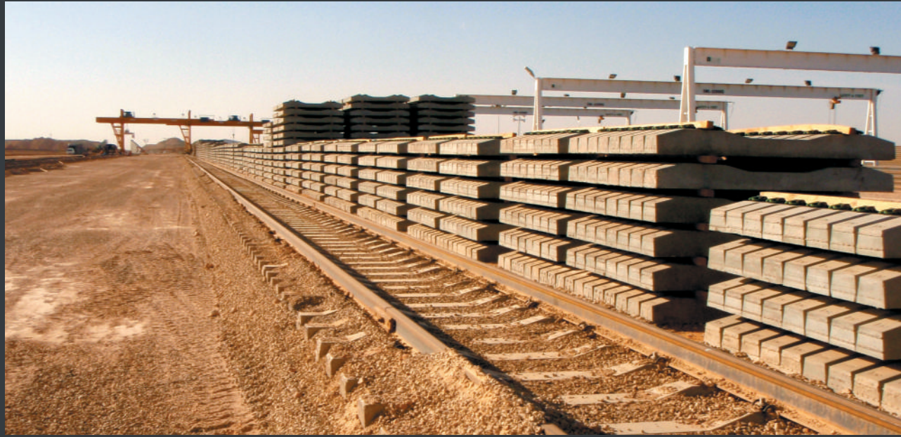
Sleepers stacking yard
