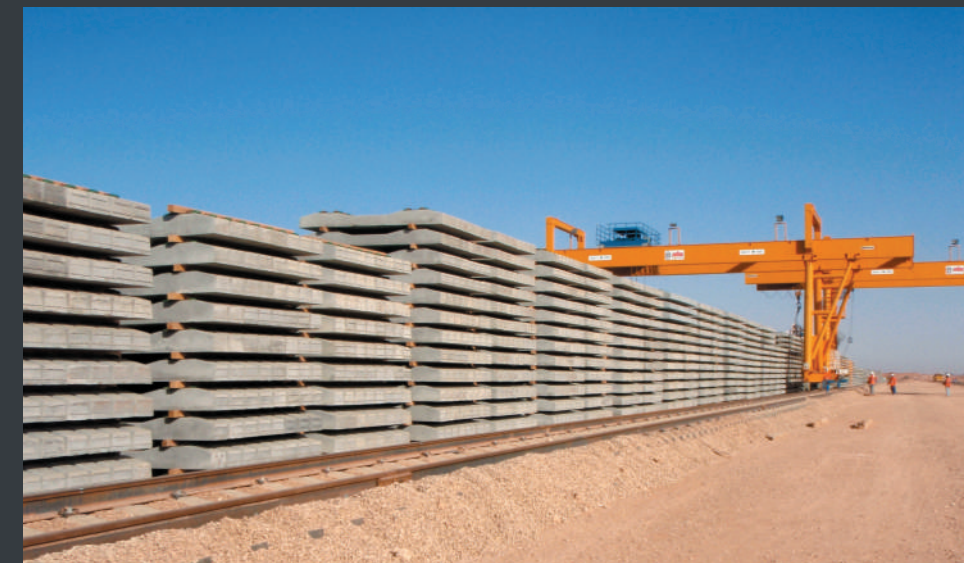
Gantry for Sleepers stacking
